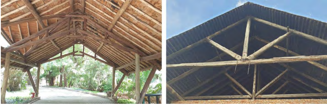
Fig. 2-2 Traditional roundwood trusses in rural areas
