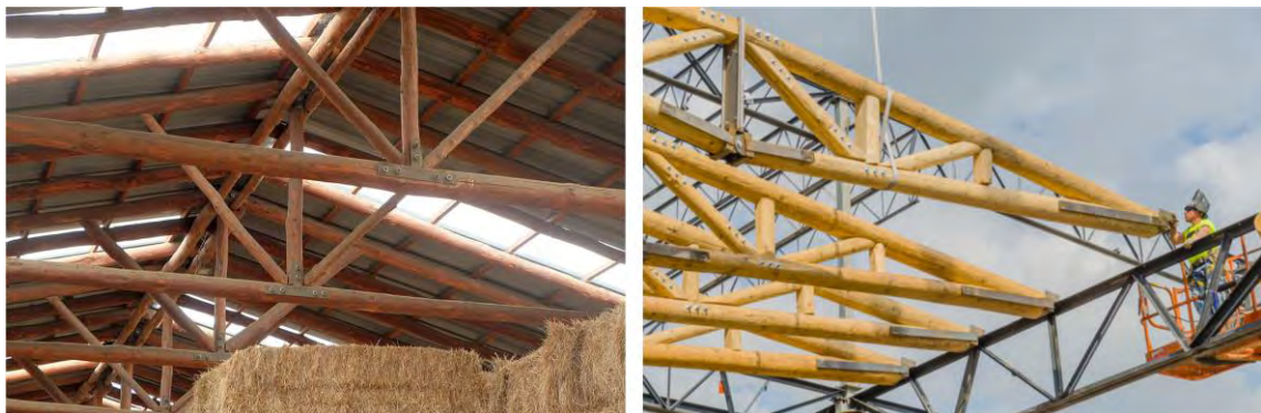
Fig. 2-3 Dowel-type connectors with steel plates for structural roundwood [with permission of the owners/authors of the pictures]
