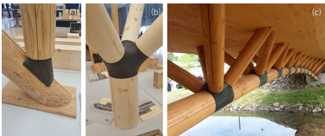
Fig. 2-14 Moulded joints composed of polymer concrete
