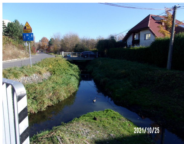
Figure A15. Wolica Canal draining rainwater from Ursynów with an intensity of 8 \text{ m}^3\text{s}^{-1} at the confluence with the Służewiecki Stream (source: own).
