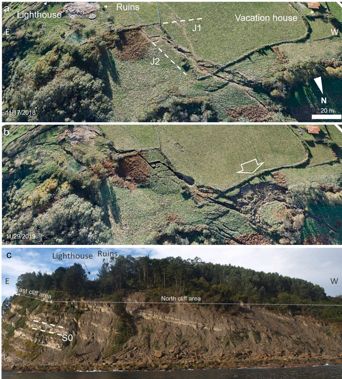
Fig. 5. Tazones Lighthouse slope evolution illustrated on the drone flight imagery of: a. 2018 and b. 2019. Main families of joints (J1 and J2) are shown. A surficial planar slide is indicated by the arrow. c. View of the cliff from the sea showing some detached metric-sized blocks and trees.
