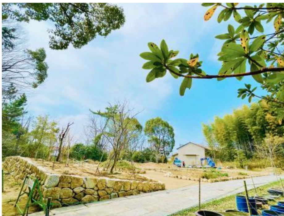
Figure 6. Herb garden under construction at Toshodaiji Temple. (Authors’ original photograph).
