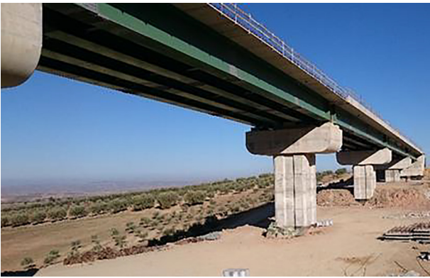
Fig. 2. General view of the composite steel-concrete viaduct
