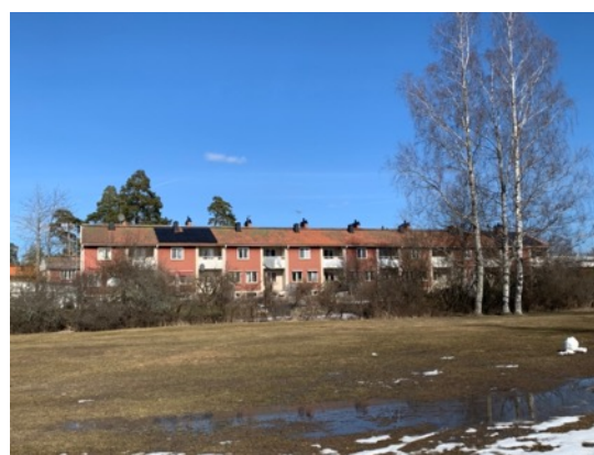
Figure 18: Apartments complex in Norby.
