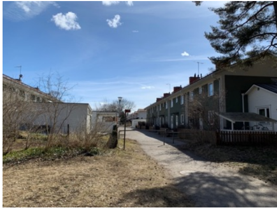
Figure 19: Row house in Norby.
