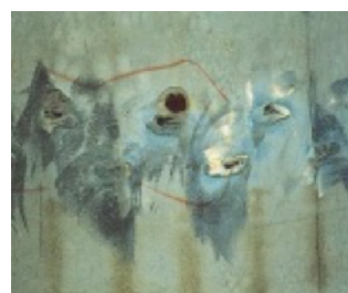
FIGURE 8. Mechanical Damage [Tang &amp; Goodwin 2001]
