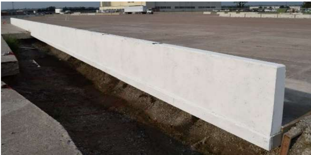
Figure 4: Bridge Deck mock-up (Akintunde et al. 2021)
