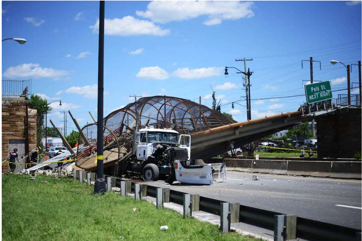
Figure 2: Lane Place Bridge Collapse
