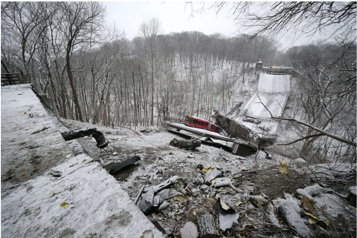
Figure 1: Frick Hallow Bridge Collapse
