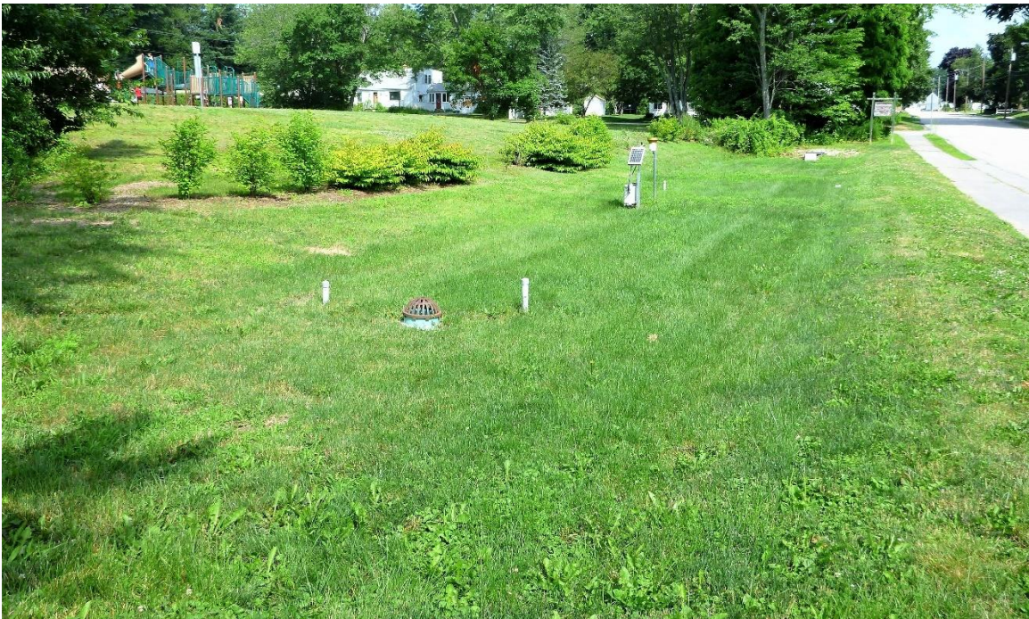
Figure 13: Horne St. bioretention system viewed from the South showing the high-flow bypass and two wells with P41 and P42 pressure transducers.
