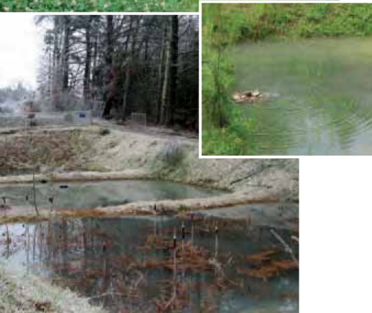
Subsurface gravel wetlands do an exceptional job of treating stormwater quality and managing water quantity. The design for the gravel wetland pictured above is helping New Hampshire's Department of Transportation meet Total Maximum Daily Load (TMDL) standards for numerous transportation improvement projects.
