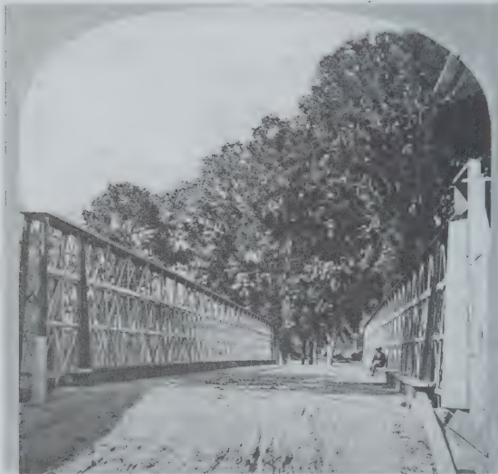
Winchester Iron Bridge, looking West.
