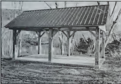
Built under direction of Lee Gamache
