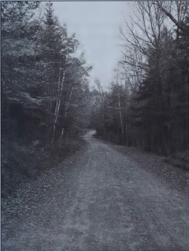
Section of Tug Mountain Road upgraded to Class V
