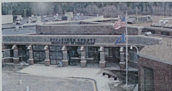
Strafford County Department of Corrections/Jail New Addition 2005
