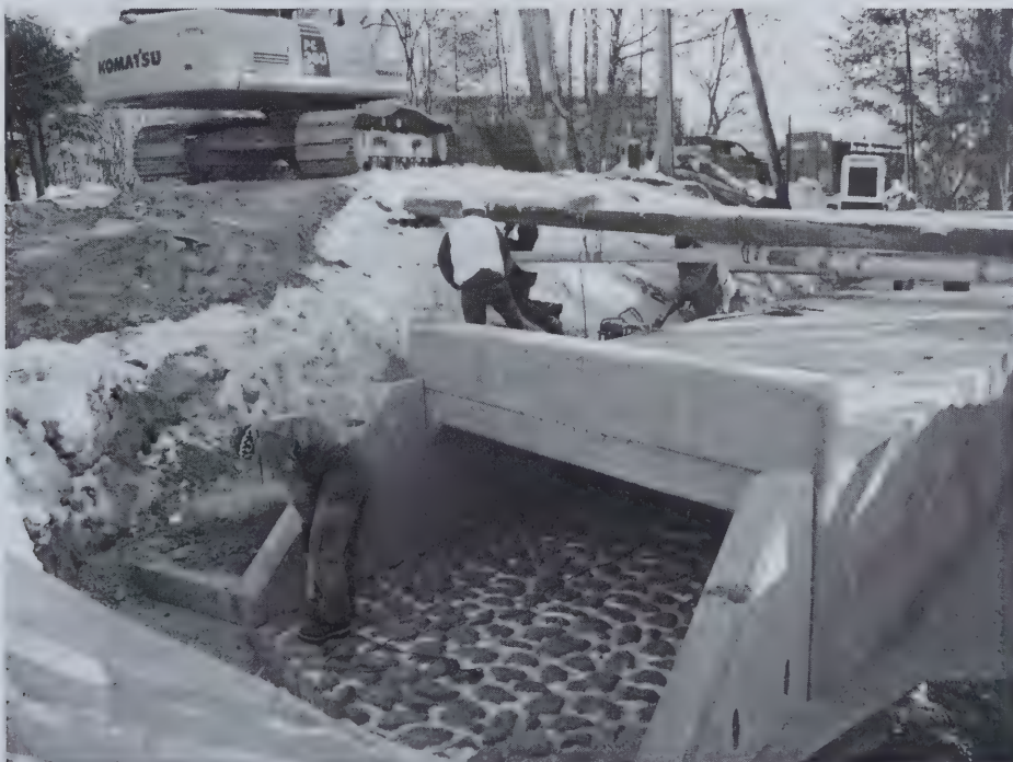
Industrial Drive Culvert Installation
