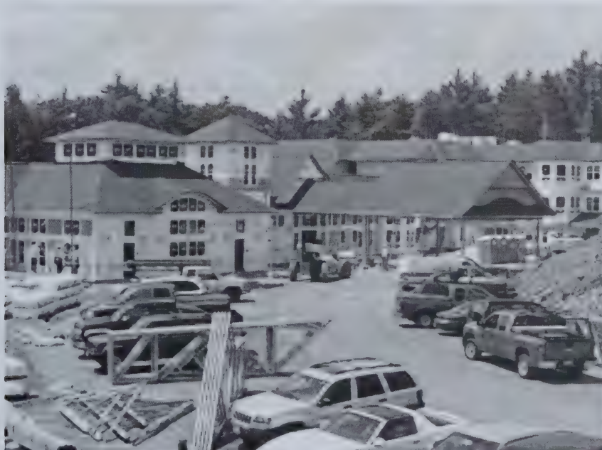
Construction at the Boulders
