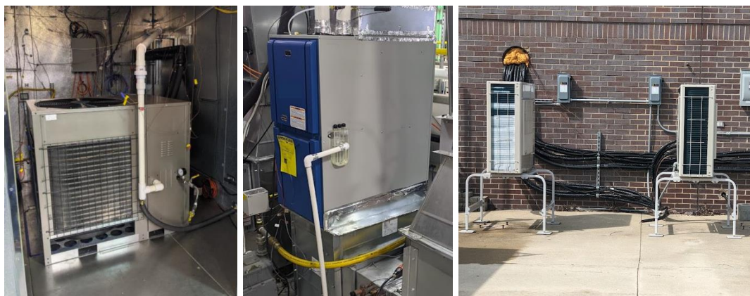
Figure 1. Examples of residential forced-air heating appliances rated to three different standards: Fuel-fired Heat Pumps – ANSI Z21.40.4 (L), Furnaces – ASHRAE 103 (M), Electric Heat Pumps – AHRI 210/240 (R)
