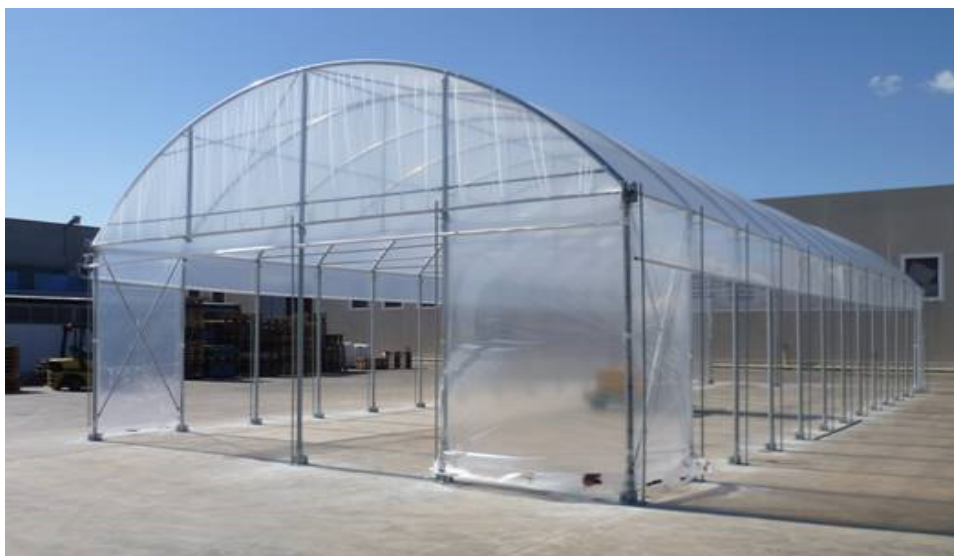
Figure 1. Greenhouse structure built for the composting tests.
