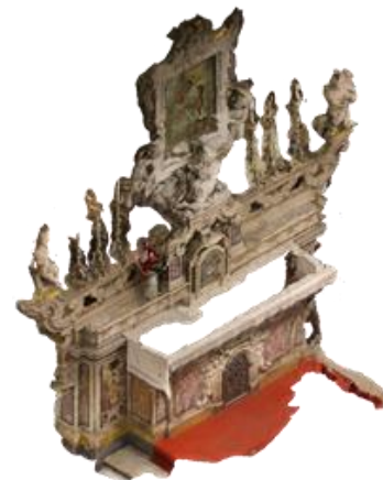
Figure 3. Altar of cathedral crypt, proof of the 3D model (obtained by Agisoft Photoscan software)
