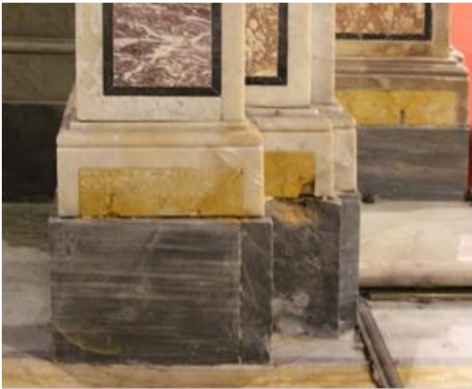
Figure 4. Altar in the crypt of the St. Sabino's cathedral: detachments and losses of stone material
