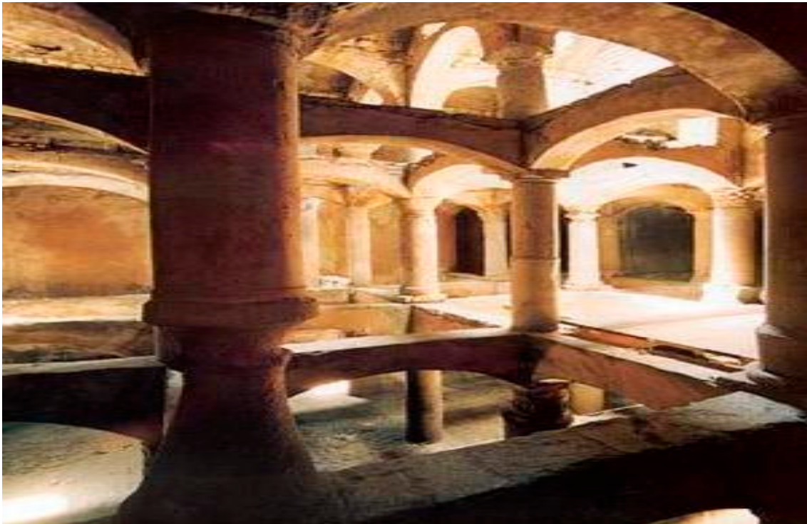
Figure 5. El-Nabih Roman cistern beneath Alexandria (Egypt), supported by a three-floor structure. In Alexandria, so far more than hundred ancient cisterns have been identified [25].
