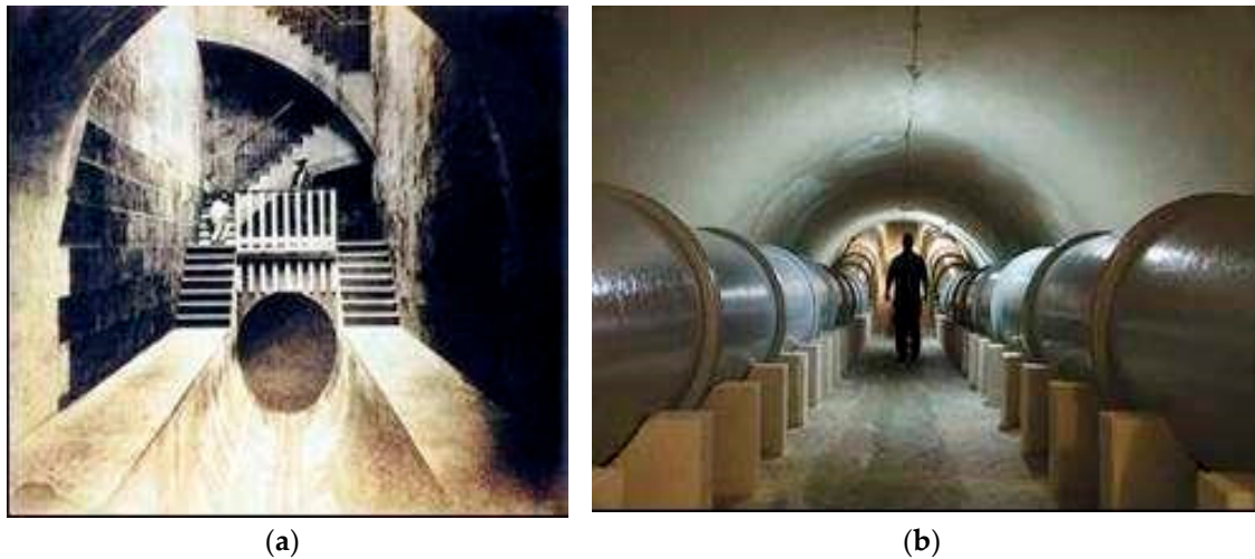
Figure 26. Alvear aqueduct at Havana, Cuba: (a) in 1927; (b) in 2012 [79].
