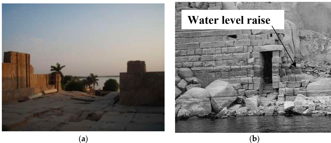
Figure 4. The Nile: (a) view from a temple bordering the river bank of the Nile (photo by M. Salgot); (b) walls of a temple located near the river bank of the Nile, where the mark of the water level raise during the river floods coincides with a passage allowing the direct water flow to the underneath temple’s aqueduct [24].
