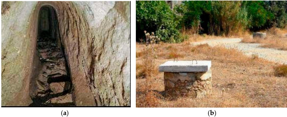
Figure 12. Roman underground aqueduct in the Aegean island of Rhodes, Greece: (a) part of the underground tunnel; (b) aligned shafts at the ground surface (photos by A. N. Angelakis).
