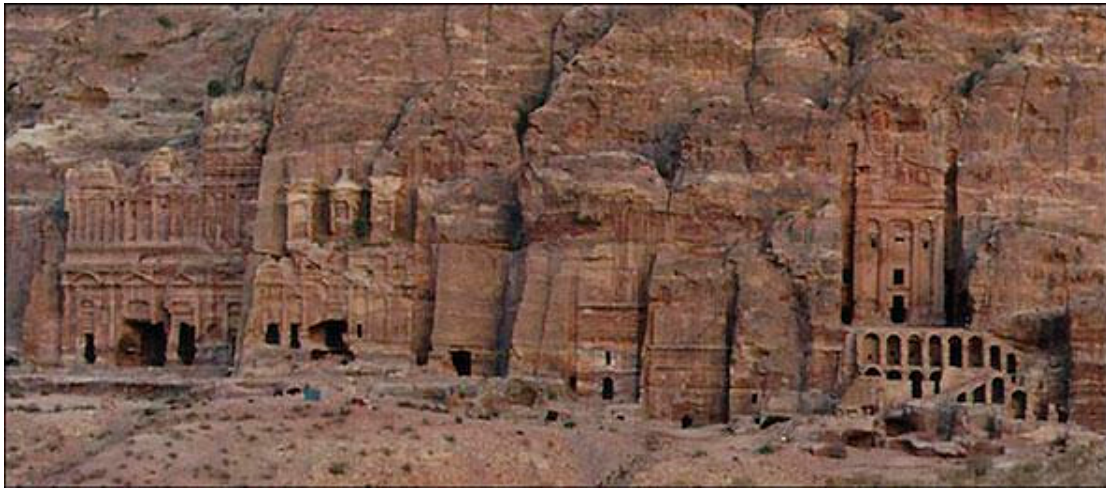
Figure 16. Carved cave structures in the Petra city, endowed with subsurface water storage function [57]. Note the keyhole shapes at the tomb entrances and the whitish effect of salt-laden water wicking into sandstone from the upper ground [59].
