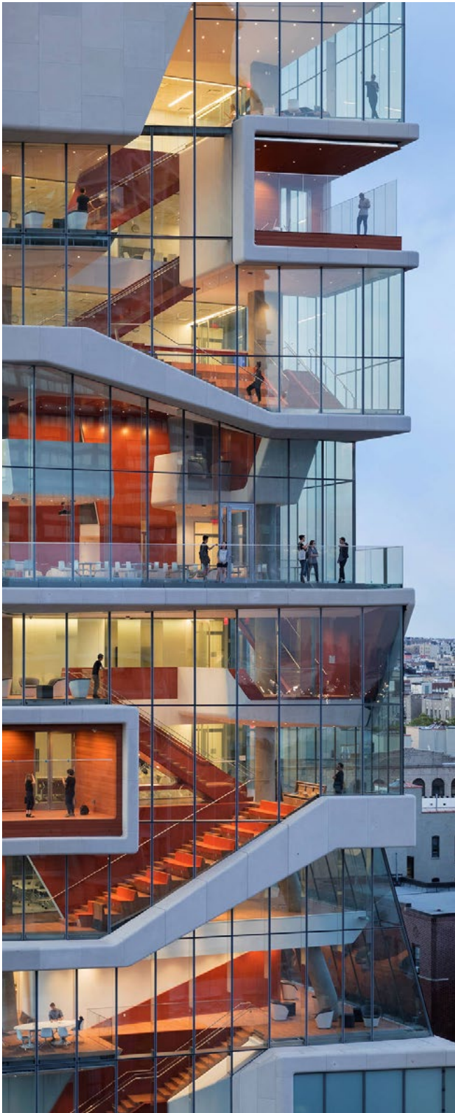
FIG. 53 “Study Cascade” of Vagelos Education Center Columbia University, New York, designed by Diller Scofidio + Renfro (2016). Photo Iwan Baan
