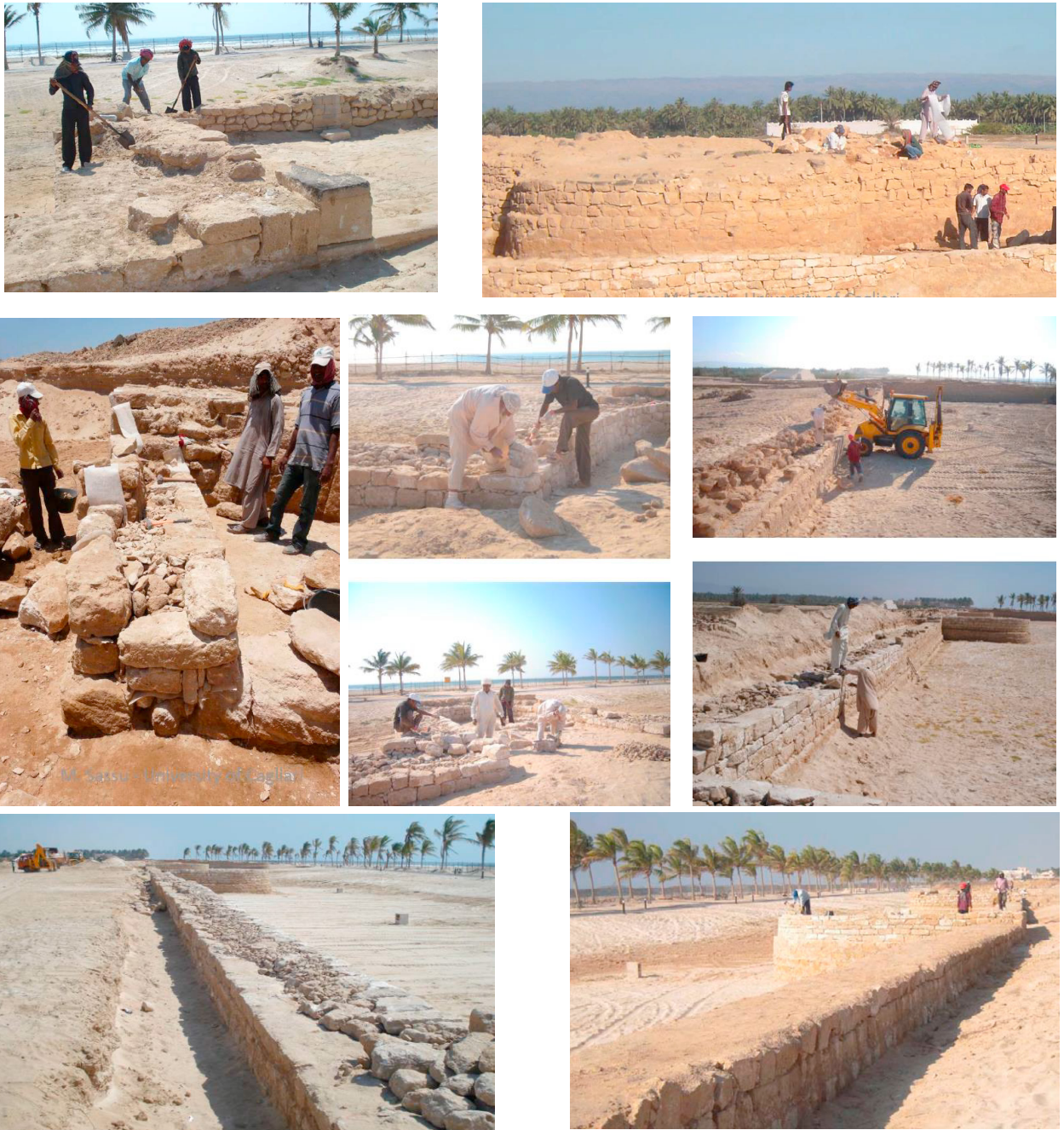
Fig. 5. Cleaning, preparation and re-construction phases in Al Balid city walls.
