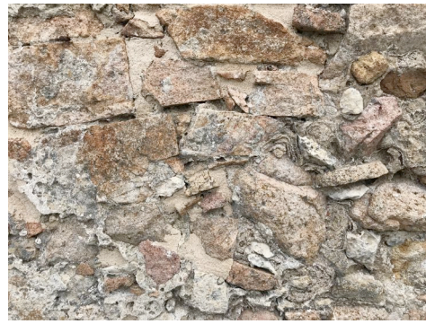
Fig. 8. Stone irregular ashlars of North side tower wall
