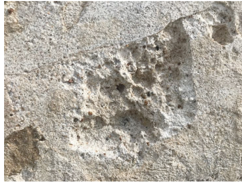
Fig. 10. Plaster mortar from West side of tower wall
