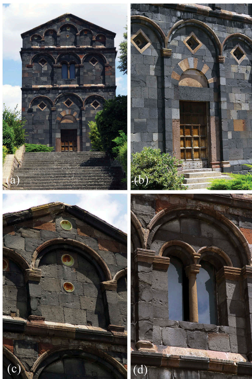
Figure 1. The San Nicola Church: (a) main façade; (b) detail on the front door of the Church, which highlight the use of ignimbrite facies of different colors, from red-rose to greyish to blackish; (c) central arch detail under the roof of the Church, with evident loss of cohesion, material detachment from the cornice, corbels, and capitals, and exfoliation in pilaster strips; and (d) details of the mullioned window, which evidence the decohesion, exfoliation, and flaking of the ashlars under the main cornice of the façade.
