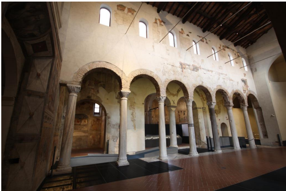
Figure 1. The side chapels: the current situation (top) and the project with a photo-insertion of the ramps (bottom).
