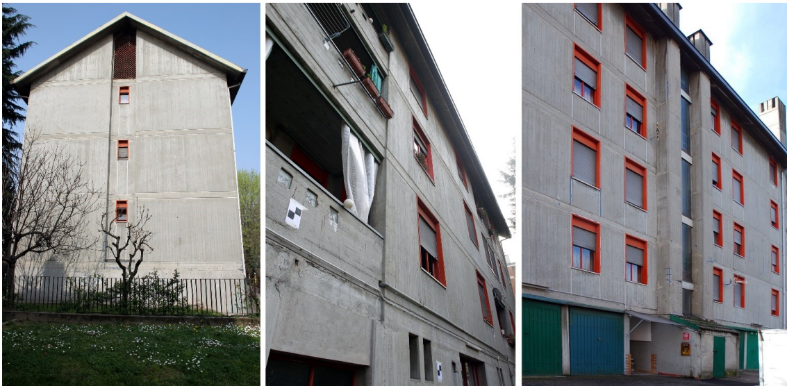
Figure 3. Existing façades of the Italian demo building.
