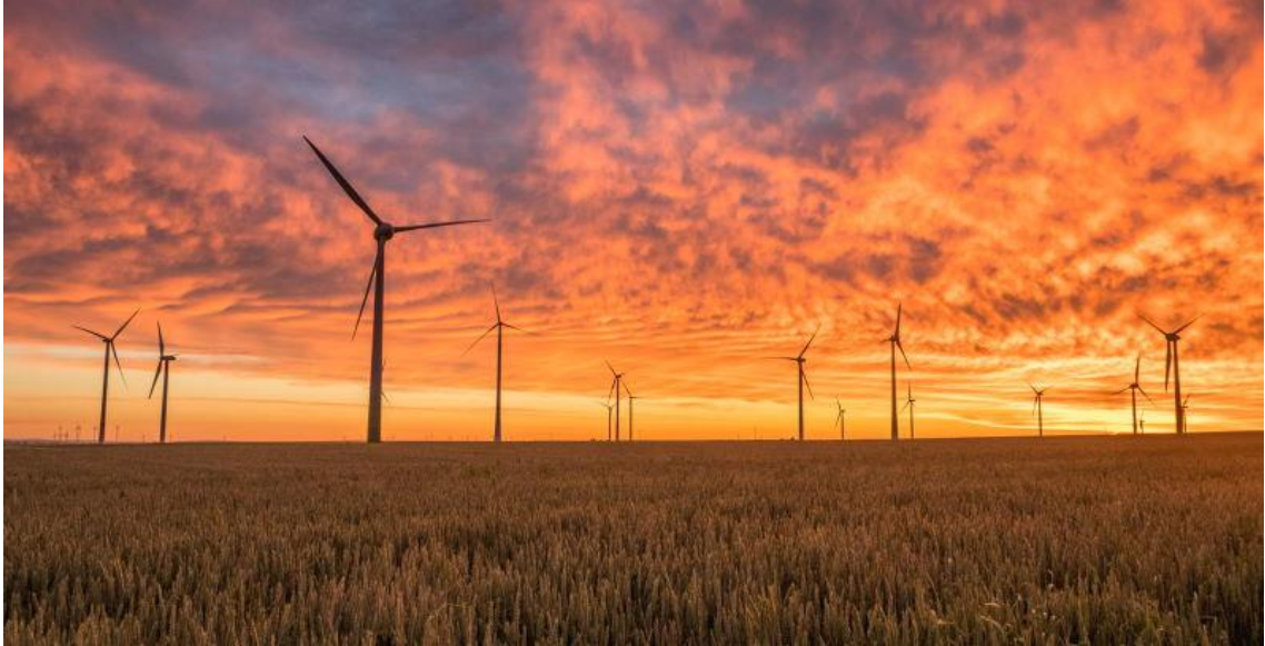
Figure 6. Example of a Wind Farm (Balkan Green Energy News, 2020)
