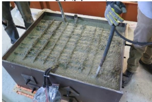
(f) Concrete placement
