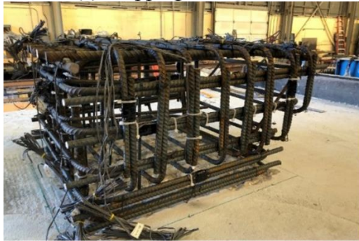
(c) Strain gauges on reinforcement
