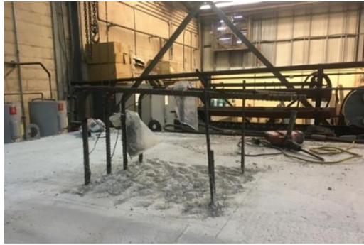
(a) Chipping the interface
