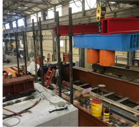
(b) Loading frame during Installation
