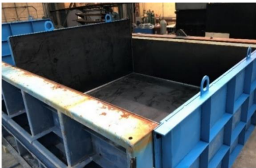
(a) Bottom soffit and side forms
