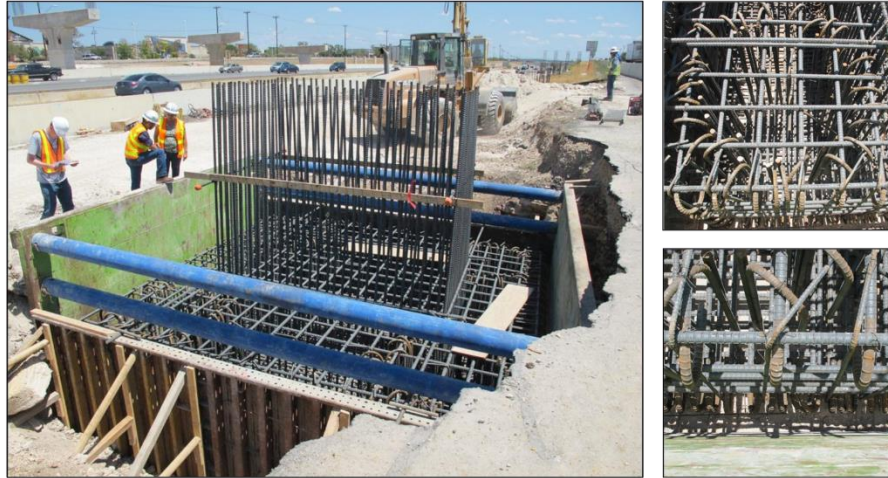
Figure 1.1 Congested reinforcement cage (footing construction at US-281 and Loop 1604 interchange)
