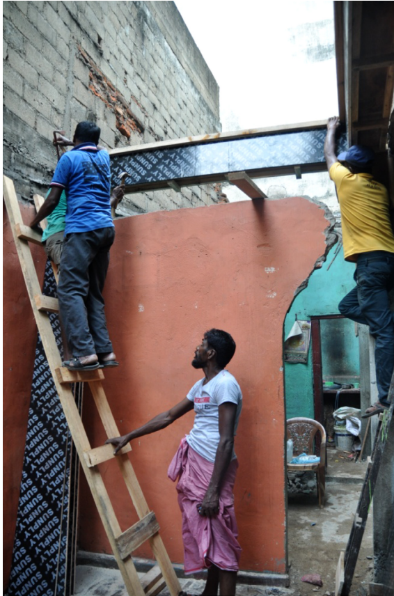
Figure 19 Self-build Construction of Structural Units, September 2017
