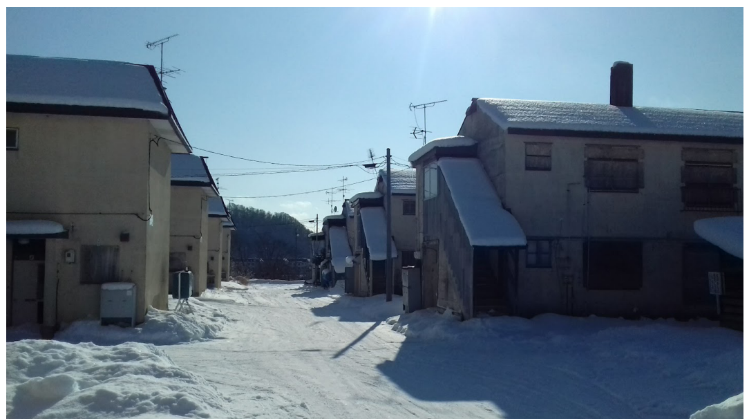
Figure 7. Former coal workers’ housing in Shimizusawa, Yubari
