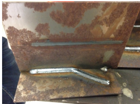
Fig. 2 Misalignment of the weld without arc sensor
