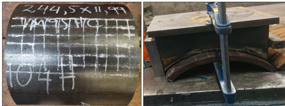
Figure 7. 1 - Measuring (left) and welding of the C-section on the adapter (right)
