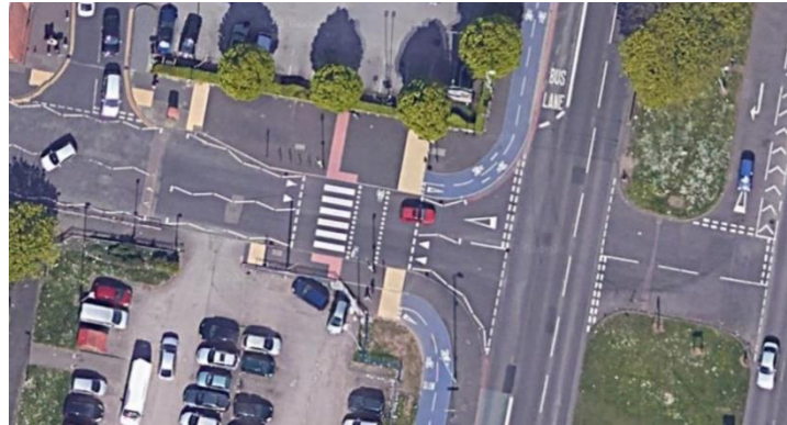
Figure 2: Milton St./A34, Birmingham
