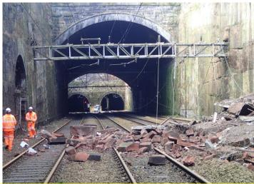
Fig.2: Debris lying on the track within a railway cutting, near Liverpool Lime Street station, UK. Note the potential for a catastrophic incident to occur if a service train had been passing through the cutting at the time, with line speeds of 30 and 40mph. **Source:** Railway Accident Investigation Branch, 2017.
