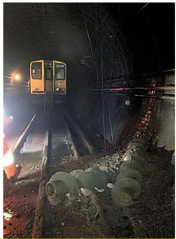
**Fig.1:** Auger and debris lying on the track of an underground railway tube tunnel after a tunnel penetration, in 2013. Note the potential for a catastrophic incident to occur if a service train had been passing through the tunnel at the time. **Source:** Railway Accident Investigation Branch, 2014.
