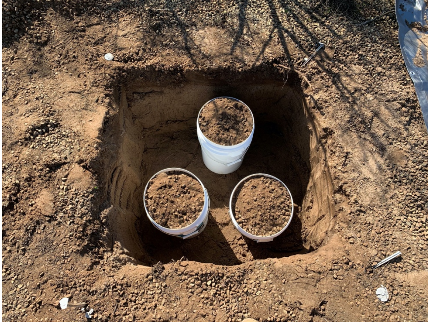
Figure 12: Filter media dug out from EBW
