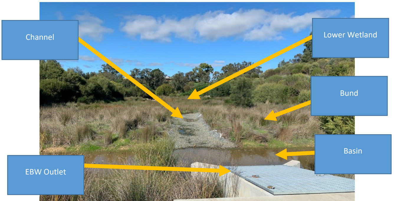
Figure 6: Channel in lower bund
