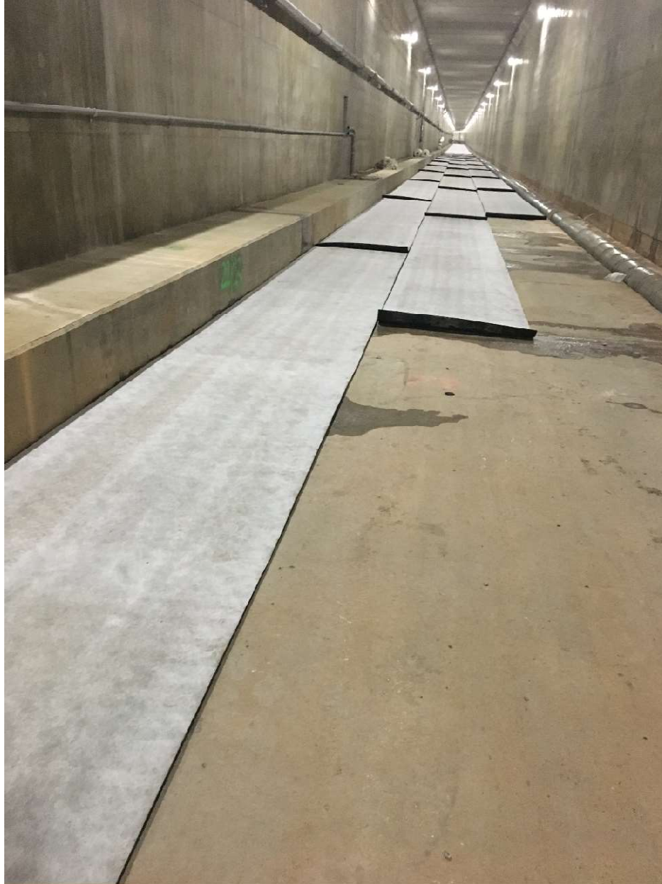
Figure 1.9.UBM during installation in the tunnel
