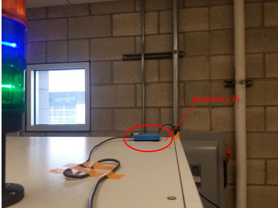
Figure 2.5: Image showing mounting location of Raspberry Pi (Top side of SLM 125)
