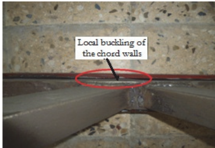
Figure 25: Left central joint failure (Experimental).
