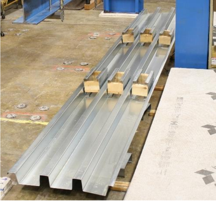
Figure 11: Stiffeners being placed inside the specimen during construction
