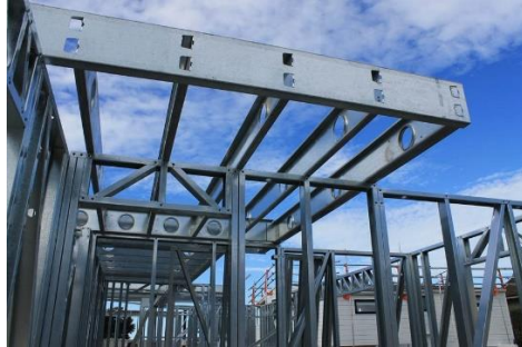
Figure 1: CFSCB as the primary load-carrying members [8]
