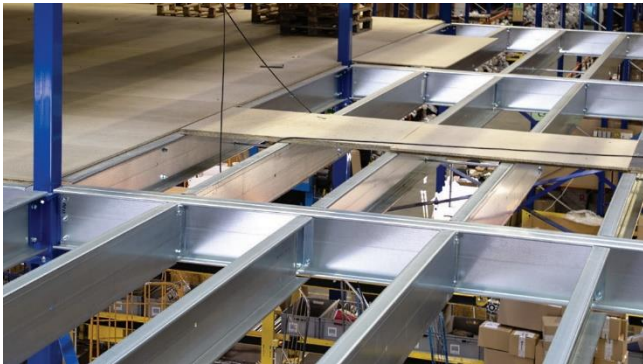
Figure 2: Composition of the floor structure (identical profile depth of primary and secondary beams) [1]
