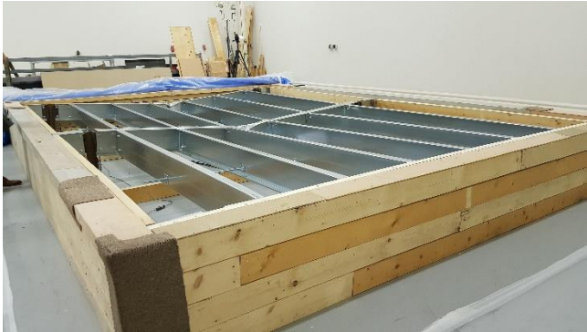
Figure 15: Collapsed load bearing structure of the mezzanine
