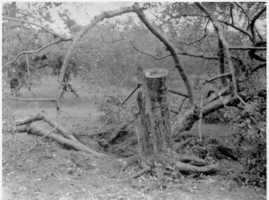
Removing the top and main branches from the tree before dynamiting resulted in a need for only 2.7 pounds of dynamite compared with 3.5 pounds for Method A.
