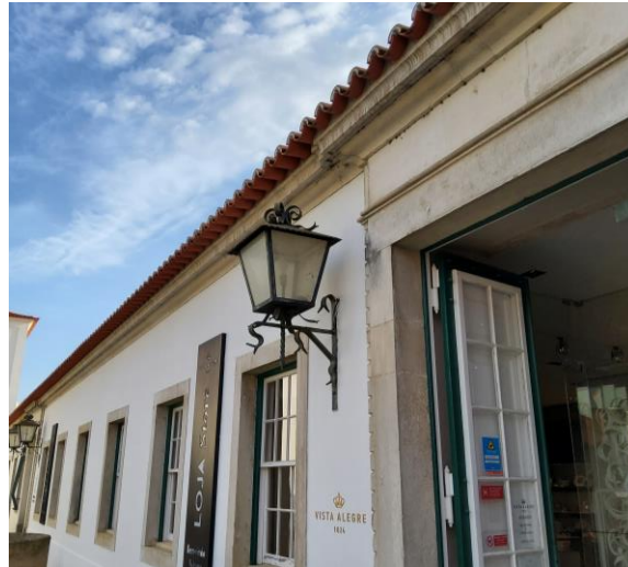
Figure 7 – The Streetlamps at the Vista Alegre compound
