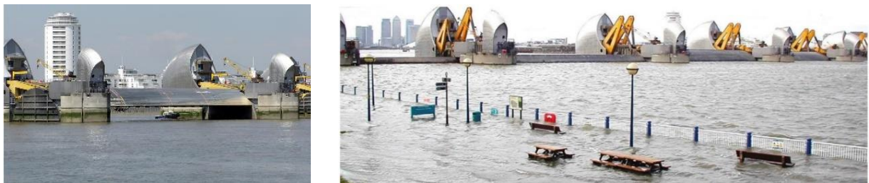
Figure 5 left. The Thames Barrier protects Central London from flooding associated with surge tides (Ramsbottom and Sheppard 2017, p.3). Figure 5 right. Surge tide at the Thames Barrier (EA 2012, p.13).
