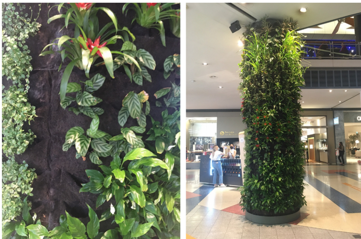
Figure 4. Continuous living wall system with felt pockets in a shopping center (Norteshopping, Matosinhos-Portugal). Credits: Cristina Calheiros.
