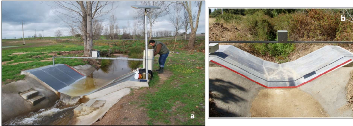
Figure 2: General view of hydrometric and water quality station.
