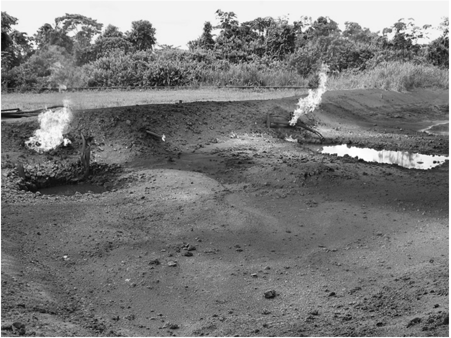
FIGURE 34 Horizontal flares burning over a partially dirt-covered, crude-oil waste pit. Photo © Amazon Watch. Used with kind permission.
