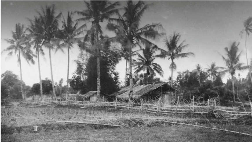
Fig. 7 Damaged Aceh houses ( source National Archive, The Hague, The Netherlands (henceforth NL-HaNA) 2.20.46_850_15)
