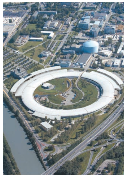
Figure 1. Artist's impression of the planned extension of the current ESRF experimental hall and the common ESRF-EMBL-ILL site.
