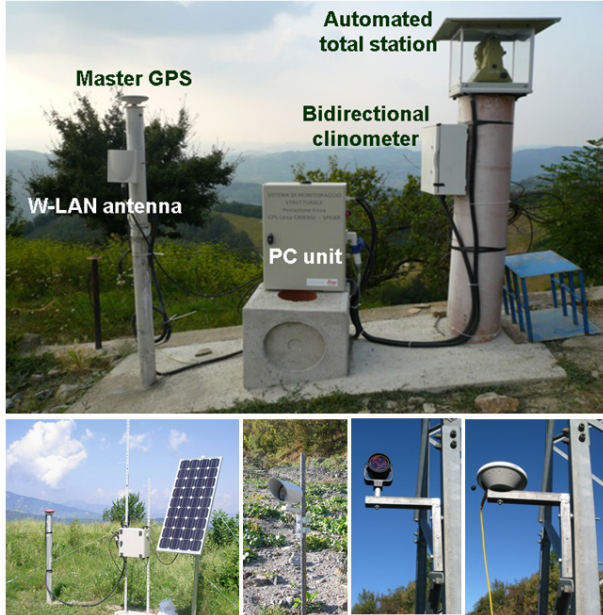
Fig. 2. Integrated monitoring system for unstable slopes: master unit at the top; below a GNSS remote site for continuous monitoring, reflectors and reference prism/GNSS
