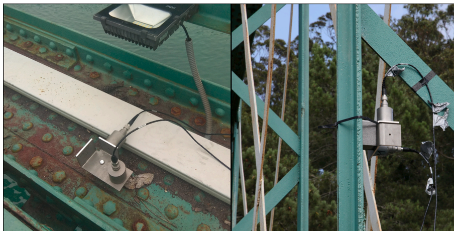
Fig. 11. Accelerometers placed on the tie girder and a vertical hanger.
