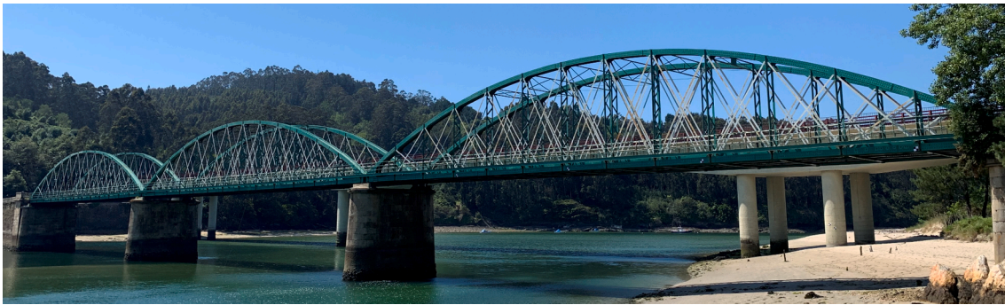
Fig. 2. Overall view of O Barqueiro Bridge.
